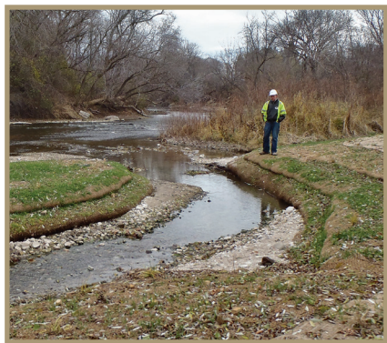
Streambank stabilization at the Taylor Wayside
