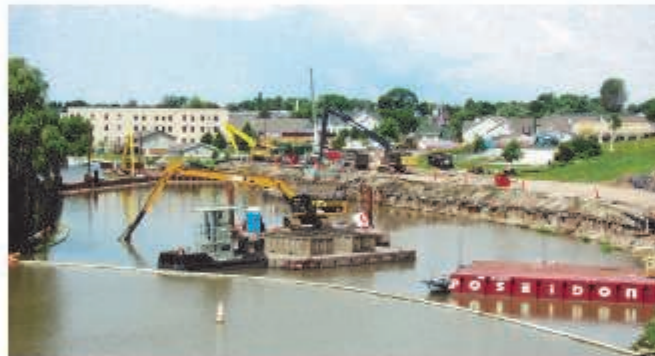
Dredging and pumping river sediment.
