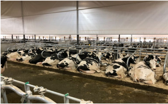
Figure 3. In a mechanically cross-ventilated barn, baffles above the stalls passively push air downward onto the cows where they lie down. Photo courtesy The Dairyland Initiative.
