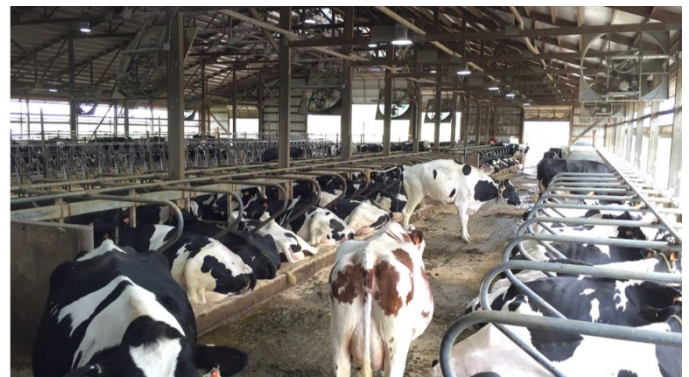
Figure 2. In a naturally ventilated barn, fans above the stalls direct fast-moving air over the cows while they rest. Photo courtesy The Dairyland Initiative.
