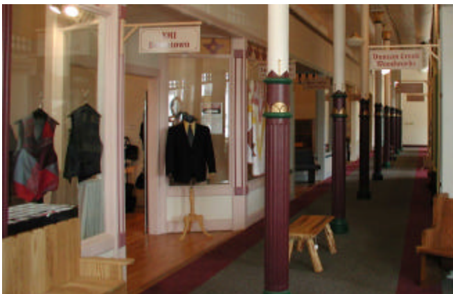
Along the Metropolitan Block's indoor "main street on main street," the first-floor metal structural supports now suggest old-fashioned light poles. Stylish interior store fronts present inviting window displays to the central hallway.
