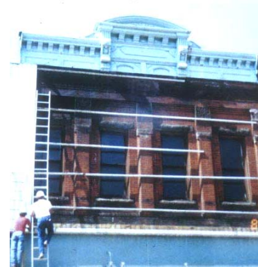
These photos from Chippewa Falls, WI show the impressive detail that was long-concealed by an inappropriate "slipcover".
