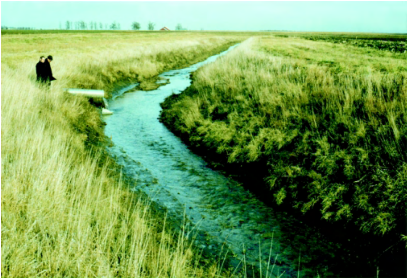
Figure 14–18 Main drain with spoil banks spread
