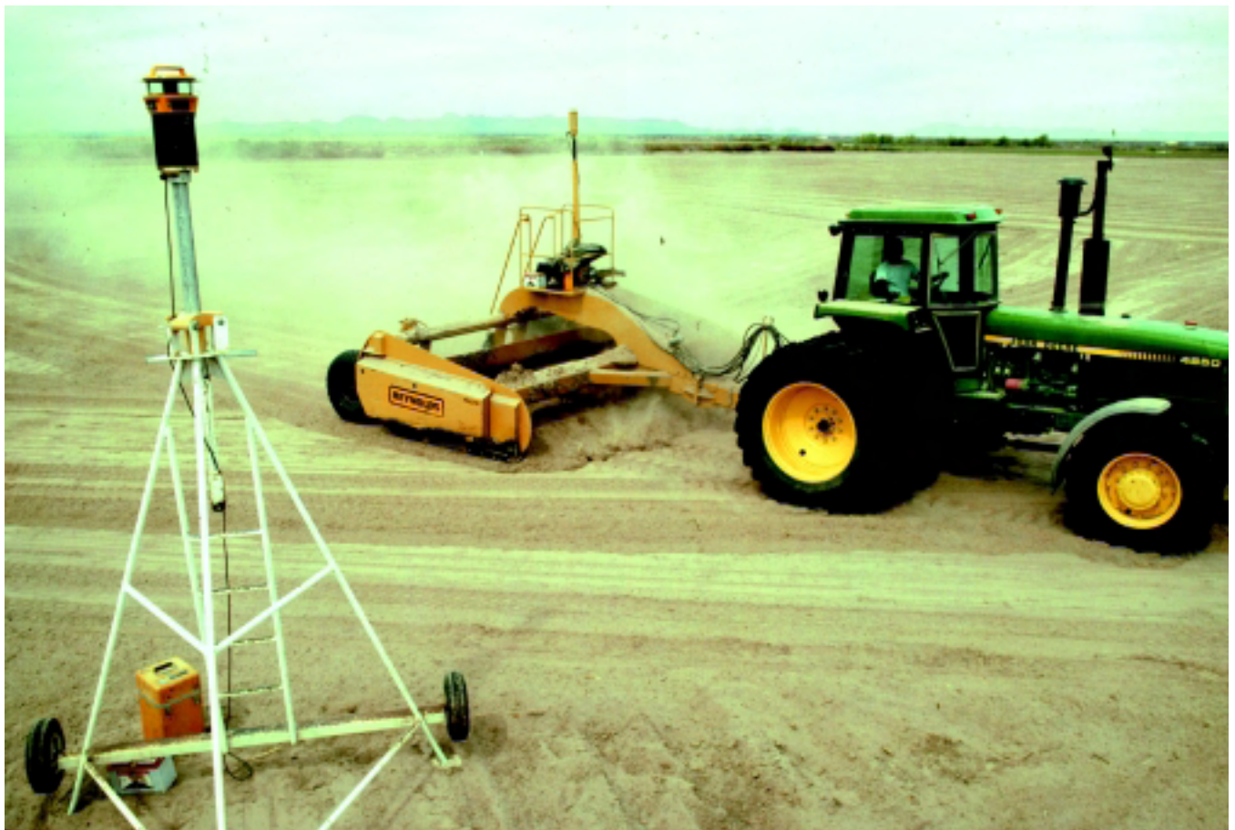
Figure 14-9 Earthmoving scraper with laser grade control
