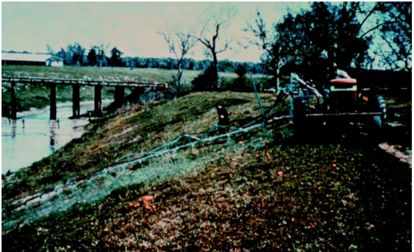
Figure 14–21 Application of chemicals for side slope weed control
