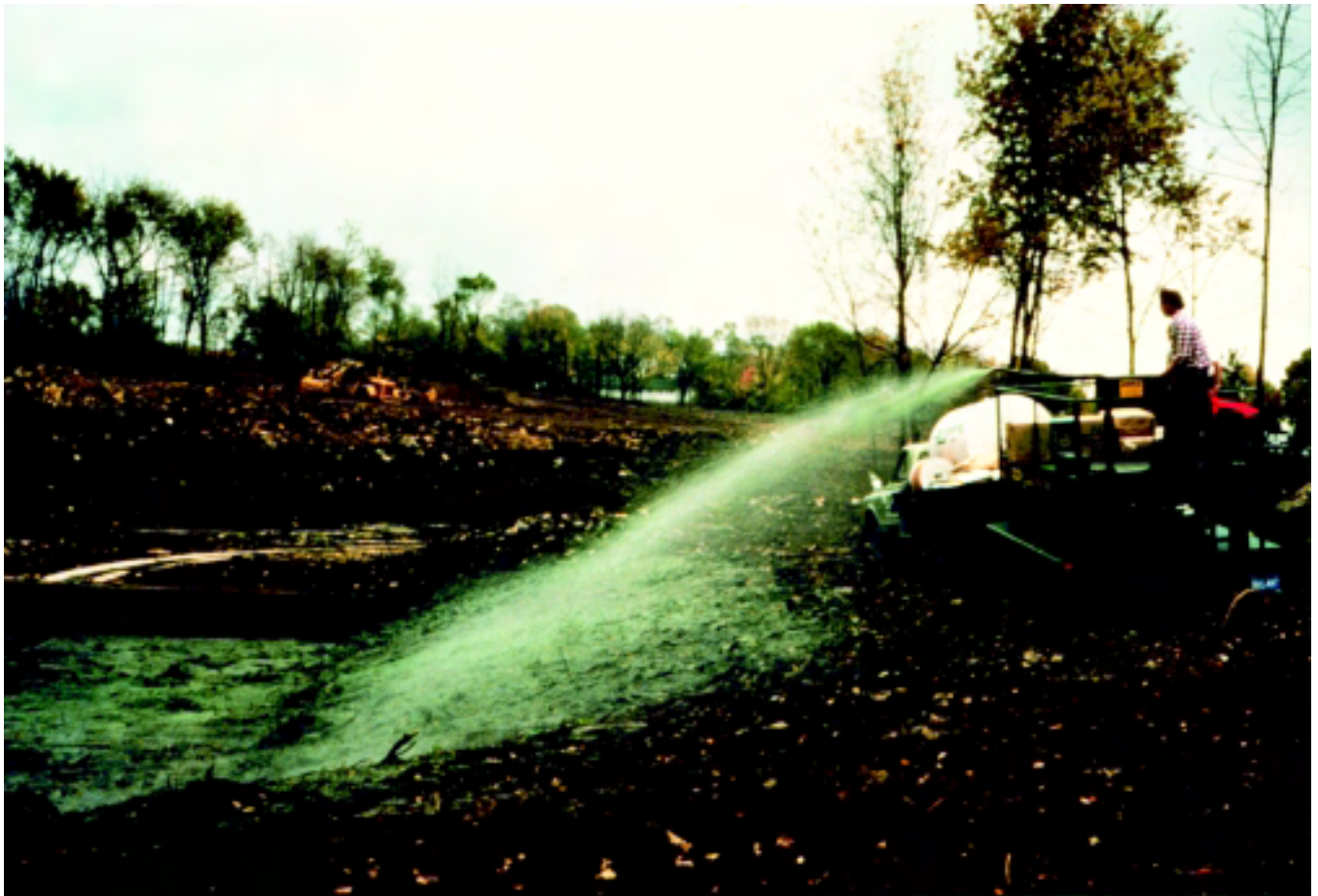
Figure 14-19 Seeding newly constructed drain
