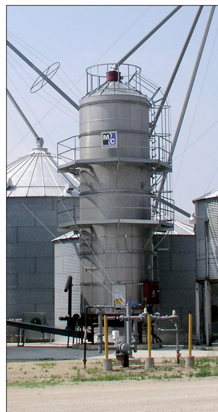
Figure 2: Tower cross-flow dryer. Source: Scott Sanford
