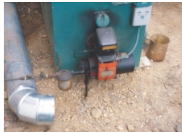
Top to bottom: Multiple boilers or furnaces increase efficiency and provide back-up insurance but increase yearly maintenance costs; Placing fuel oil tanks inside reduces midnight alarm calls due to cold oil flow problems; Extend the chimney above the peak of the greenhouse to improve draft. Add a cap to prevent back drafts; Tight greenhouses require a source of make-up air to the burner or a separate combustion air system. (Photos courtesy of John Bartok)
