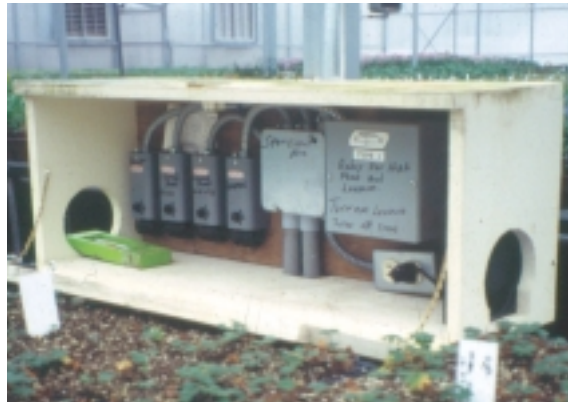
Top: If you have more than five heating units, a $300 combustion test kit will pay for itself in improved fuel efficiency; Right: Locate thermostats and sensors in an aspirated box in the plant zone.
