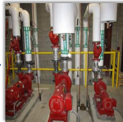
HX and Distribution Pumps to Three Facilities
