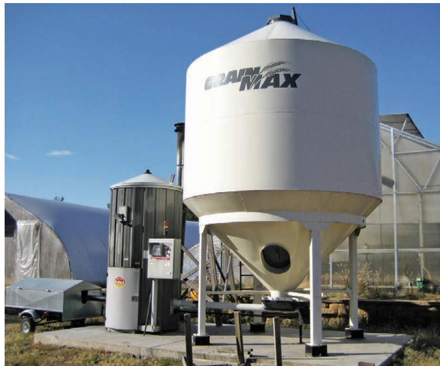
Hydronic pellet boiler with pellet storage bin.
