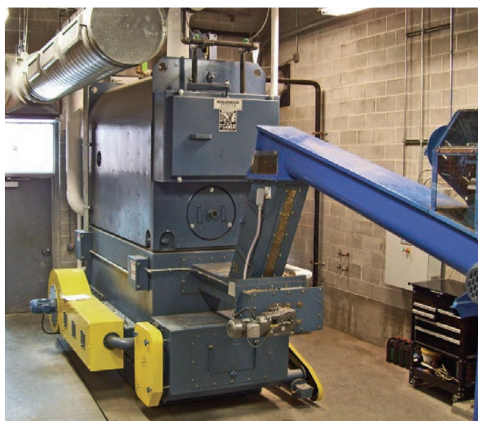
Hydronic pellet boiler with pellet storage bin.
