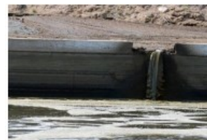
One potential hazard is someone falling into the storage and being engulfed in the manure slurry.
