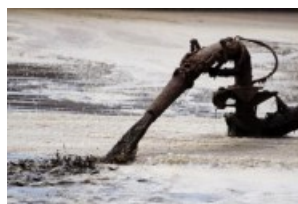
Agitation accelerates the release of hazardous gases. Employees should know the signs and symptoms of these gases.
