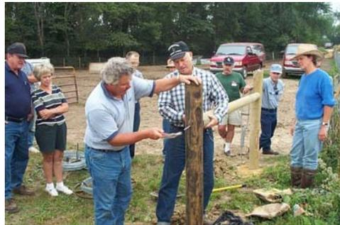
Figure 3 Attaching brace support
