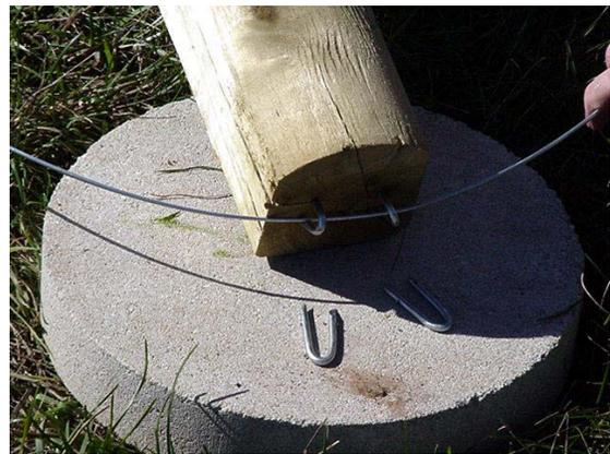
Figure 10 Attaching brace wire
