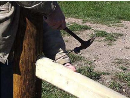
Figure 8 Attaching brace
