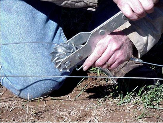
Figure 12 Tightening brace wire
