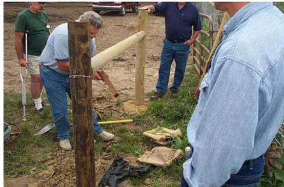
Figure 4 Tightening brace wire
