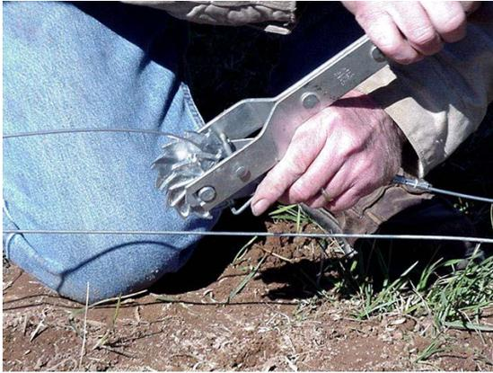
Figure 12 Tightening brace wire
