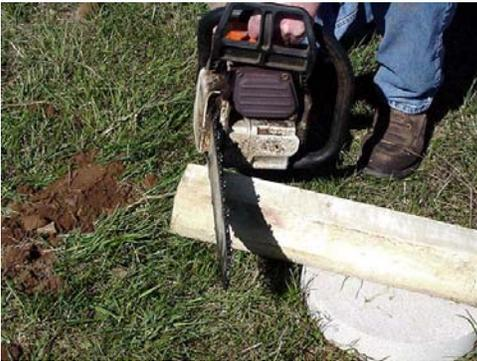
Figure 7 Cutting brace
