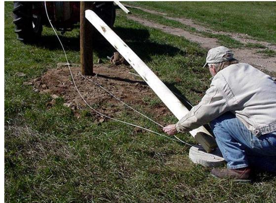
Figure 11 Adjusting brace wire
