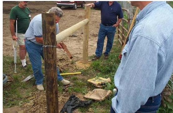
Figure 4 Tightening brace wire
