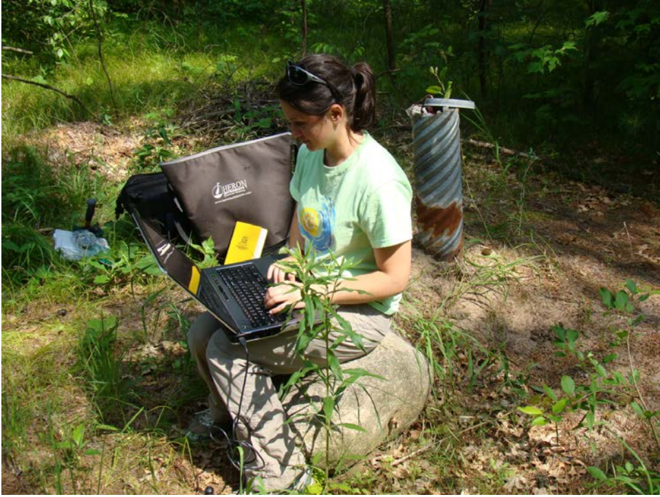
Figure 6. Installing a datalogger in an old UWSP well near the river.
