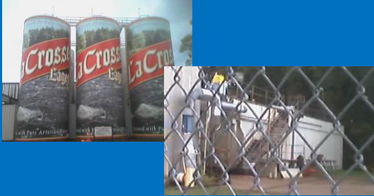
Upflow Anaerobic Sludge Blanket Reactor (UASB) City Brewery, LaCrosse, WI ca. 1982 (first UASB in USA)
