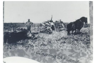
Clearing the land of stumps
