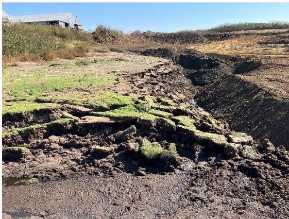
Photo 23: Clean fill being added as manure solids are removed during the 2022 NOD grant funded manure storage closure project
