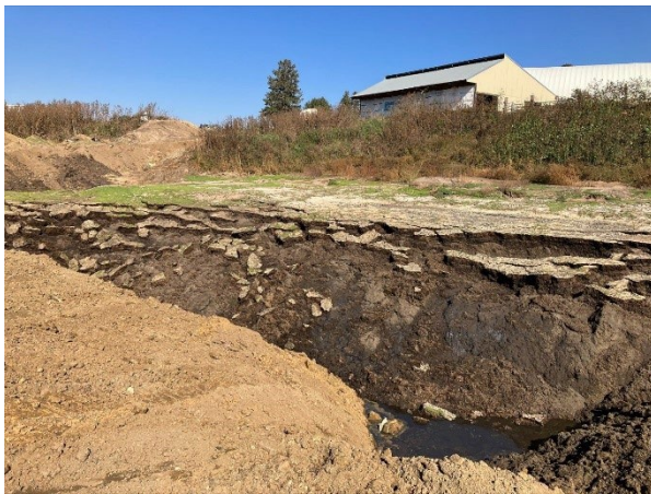
Photo 22: Clean fill being added as manure solids are removed during the 2022 NOD grant funded manure storage closure project
