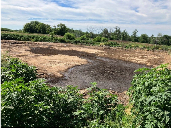
Photo 18: What the overflowing/leaking manure storage structure looked like in July 2022. NOD grant funding was used to properly close this facility.
