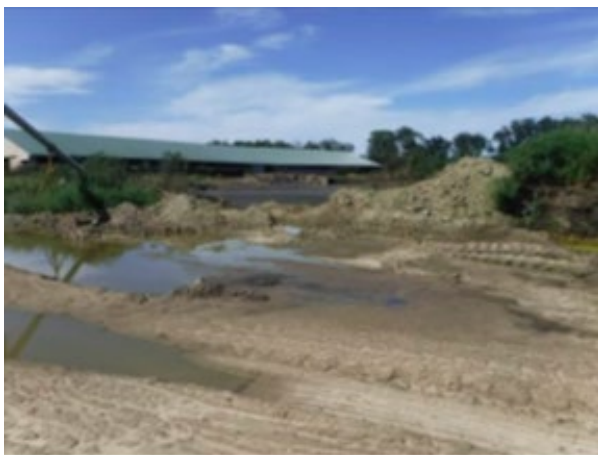
Photo 25: Overflowing manure storage to be corrected with NOD grant awarded to Dunn County in 2022
