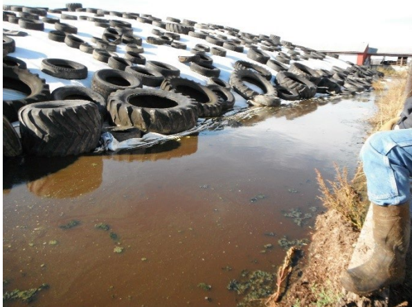
Photo 32: Runoff concerns detected during a 2017 inspection prompting investigation into animal units and nutrient management plan through an NON in 2022
