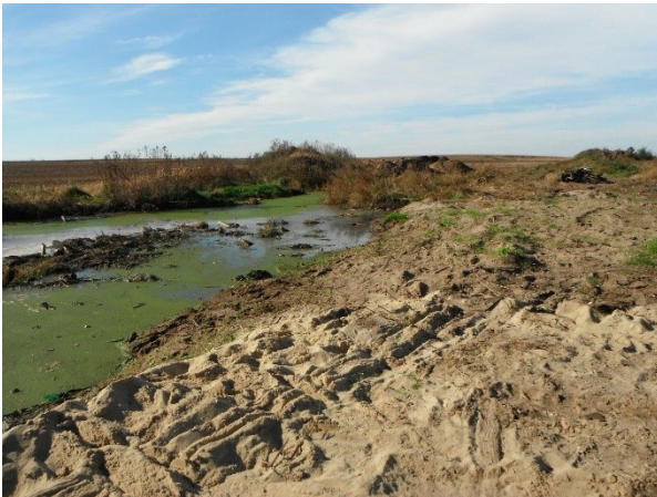
Photo 35: Runoff concerns detected during a 2017 inspection prompting investigation into animal units and nutrient management plan through an NON in 2022
