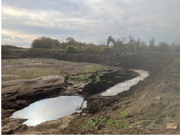
Photo 21: Manure solids being removed during the 2022 NOD grant funded manure storage closure project
