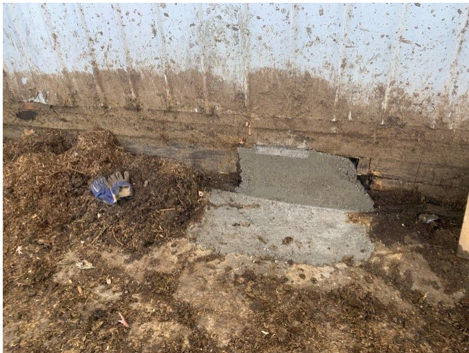
Photo 45: Pipe inlet sealed closed with concrete in 2022
