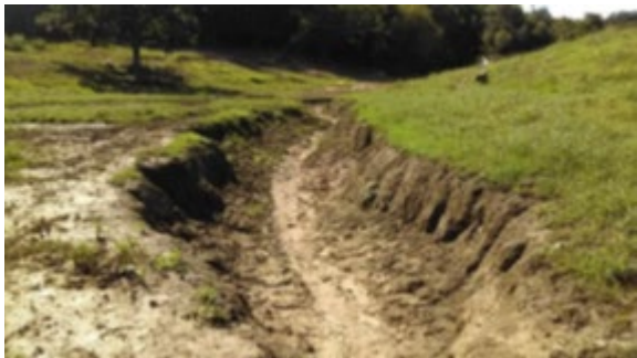
Photo 28: Intermittent stream and flow path of manure storage overflow to Lower Pine Creek. Impact to be corrected by NOD grant awarded to Dunn County in 2022
