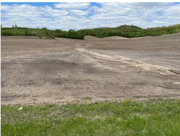
Photo 40: Field not meeting state erosion standards with pending enforcement action
