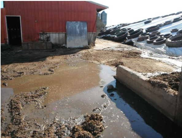
Photo 33: Runoff concerns detected during a 2017 inspection prompting investigation into animal units and nutrient management plan through an NON in 2022
