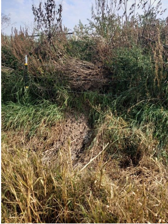
Photo 14: Manure overflowing and leaking
