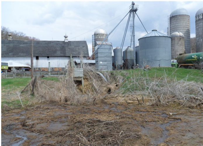
Photo 44: Underground pipe outlet discharging to wetland
