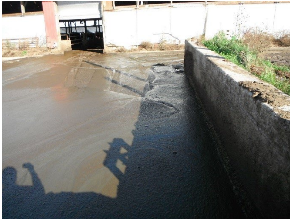
Photo 36: Runoff concerns detected during a 2017 inspection prompting investigation into animal units and nutrient management plan through an NON in 2022
