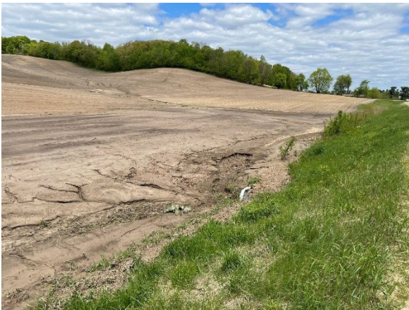
Photo 39: Sediment leaving field through road culvert
