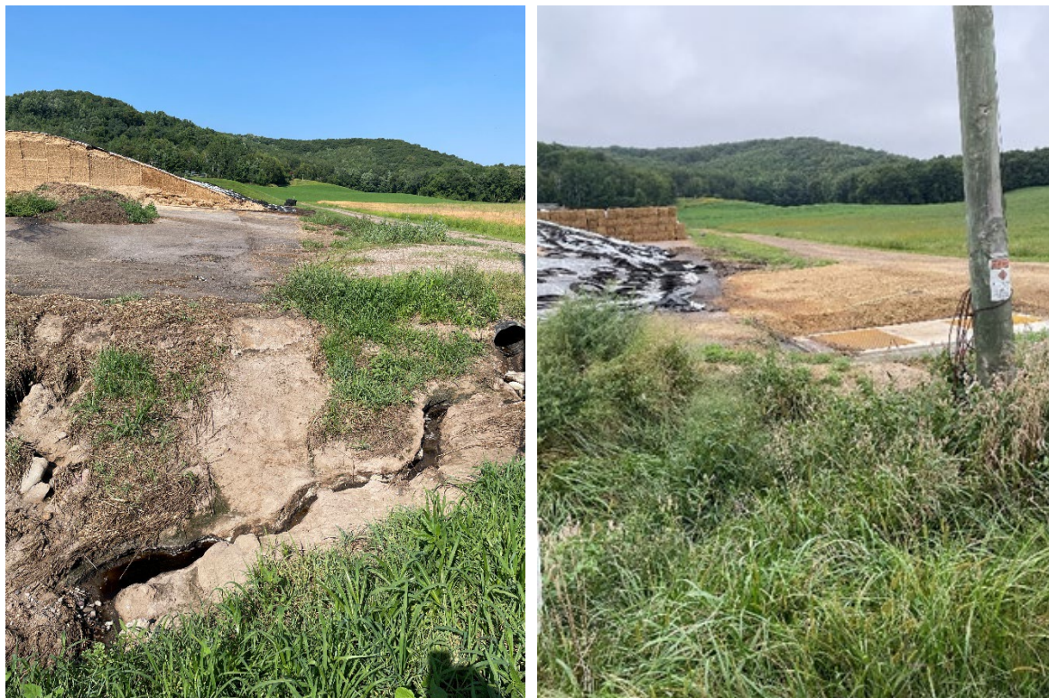
Before (left) and after (right) of Chippewa County feed leachate noncompliance resolution. Landowner's solution was to install a concrete collection tank intercepting the flow path, which can be seen in right picture.
