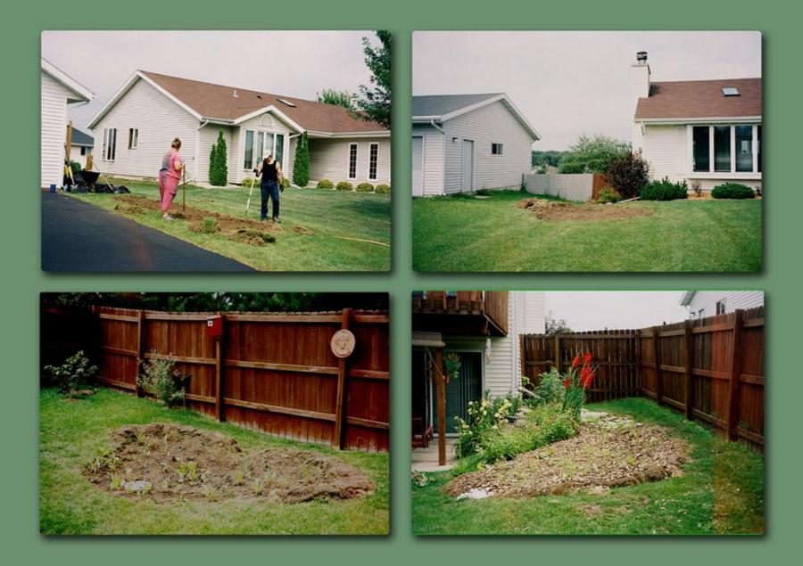
Bioinfiltration Cells -An Engineered Rain Garden
