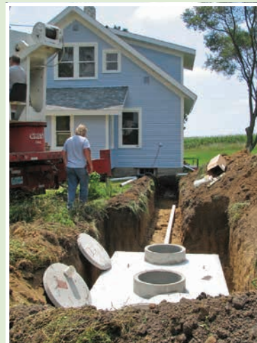
Septic System Installation
