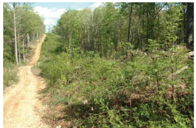
This forest road was daylighted to provide additional browse, soft mast, and nesting cover for various wildlife species. The road was graveled to prevent erosion because it receives considerable traffic from land managers.
