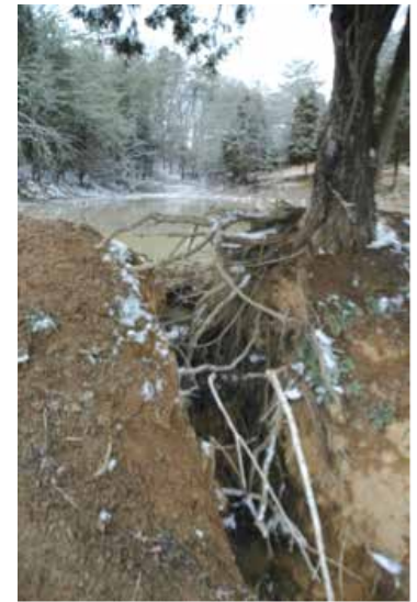
Tree roots can cause dams to fracture, leak, and eventually break.
