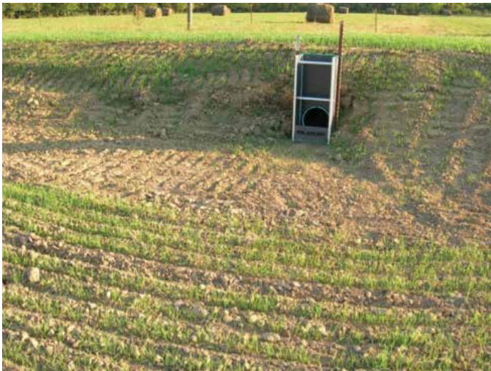
Water control structures allow manipulation of the water level in ponds and areas flooded for wildlife using a dike or levee.
