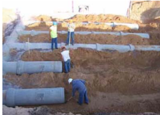
Laying the Earth Tubes.
