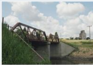
Double arch truss bridge, James River Scenic Byway, North Dakota. (Photo: Agency MABU/Annette Tait, courtesy of National Transportation Enhancements Clearinghouse. www.enhancements.org )
