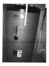
The hot water storage tank has two heat coils. The lower coil is heated by the solar panel and the upper tank is heated by the only heat source for the house: the MUNCKIN FURNACE [see below]. If the water temperature is below what is being called for, the MUNCHKIN FURNACE also functions as an 'on demand' hot water heater (see below).
