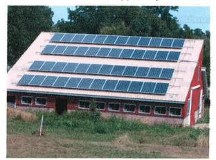
The 48 panels are arranged in two 24 unit pairs that generate 12 volt DC current that is then converted by a DC to AC converter to standard AC synchronized with Alliant Energy (Wisconsin Power and . electrical supplier. Alliant Energy assisted with the necessary permits and TIME OF USE BILLING PLAN (day time from 8 AM until 8 PM Peak Energy Cost/Payment of 20¢ per Kilo Watt and night time from 8 PM until 8 AM Off Peak Cost/Payment of 5¢ per KW.
